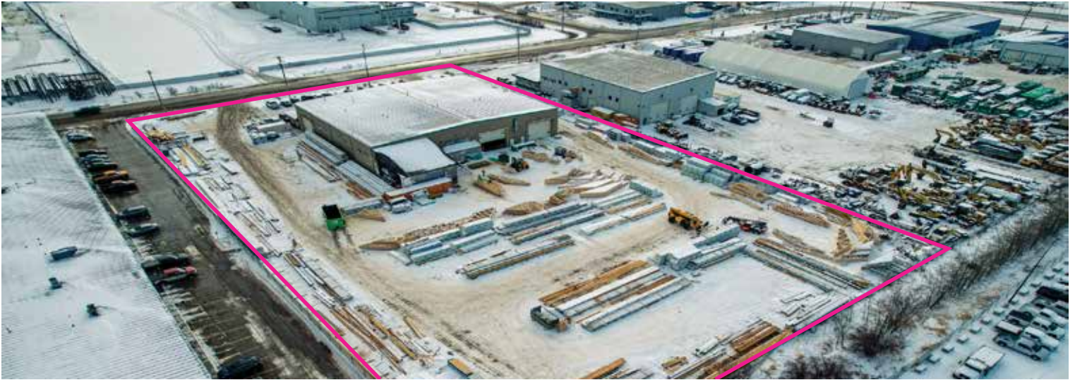
Overview of property
