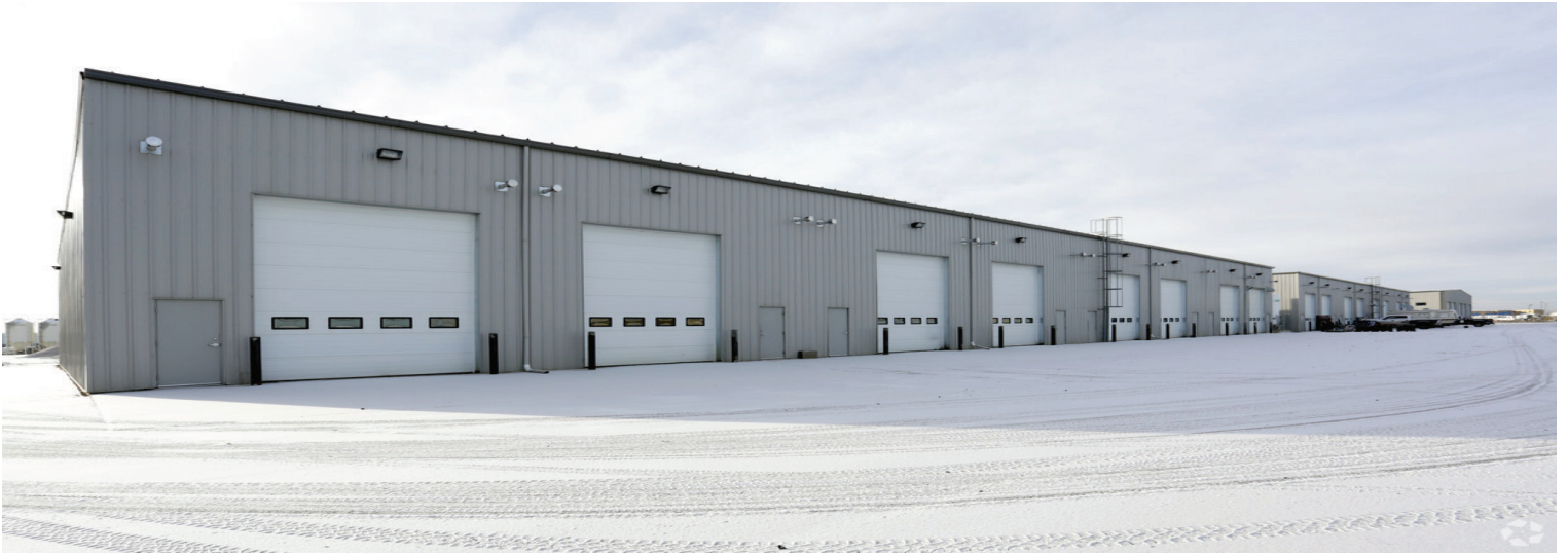
Rear grade loading door
