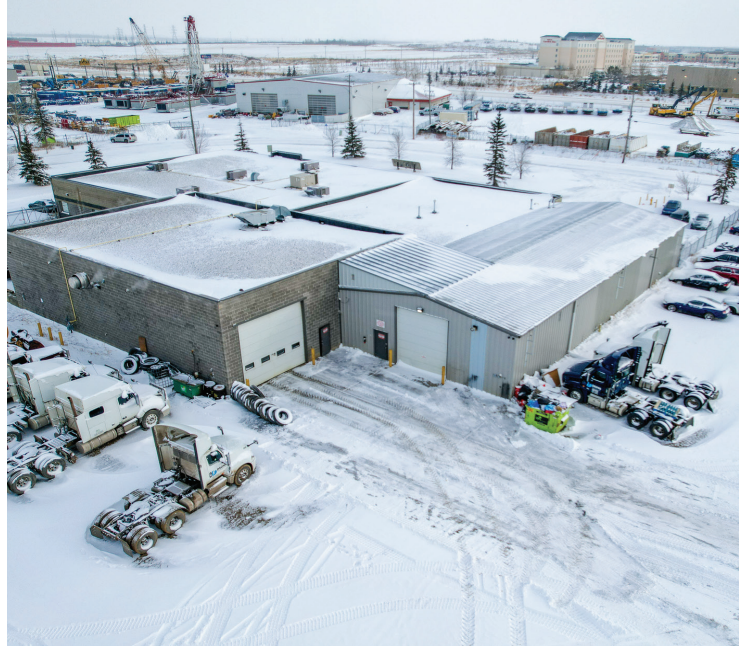
Warehouse overhead west
