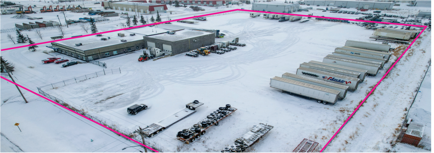
Overview of property
