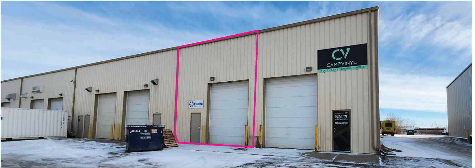
Rear grade loading door
