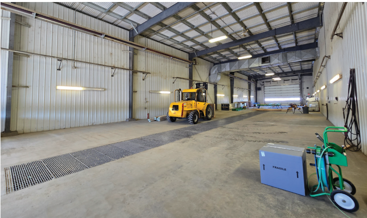
Drive-thru bay with two 24' x 16' grade doors
