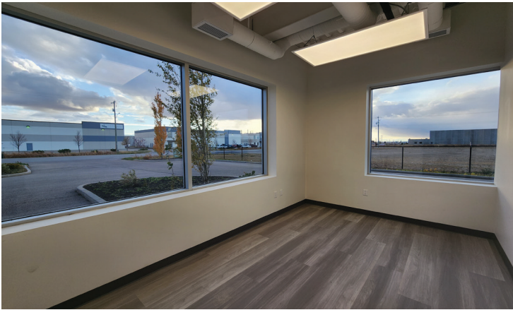
New office build-out
