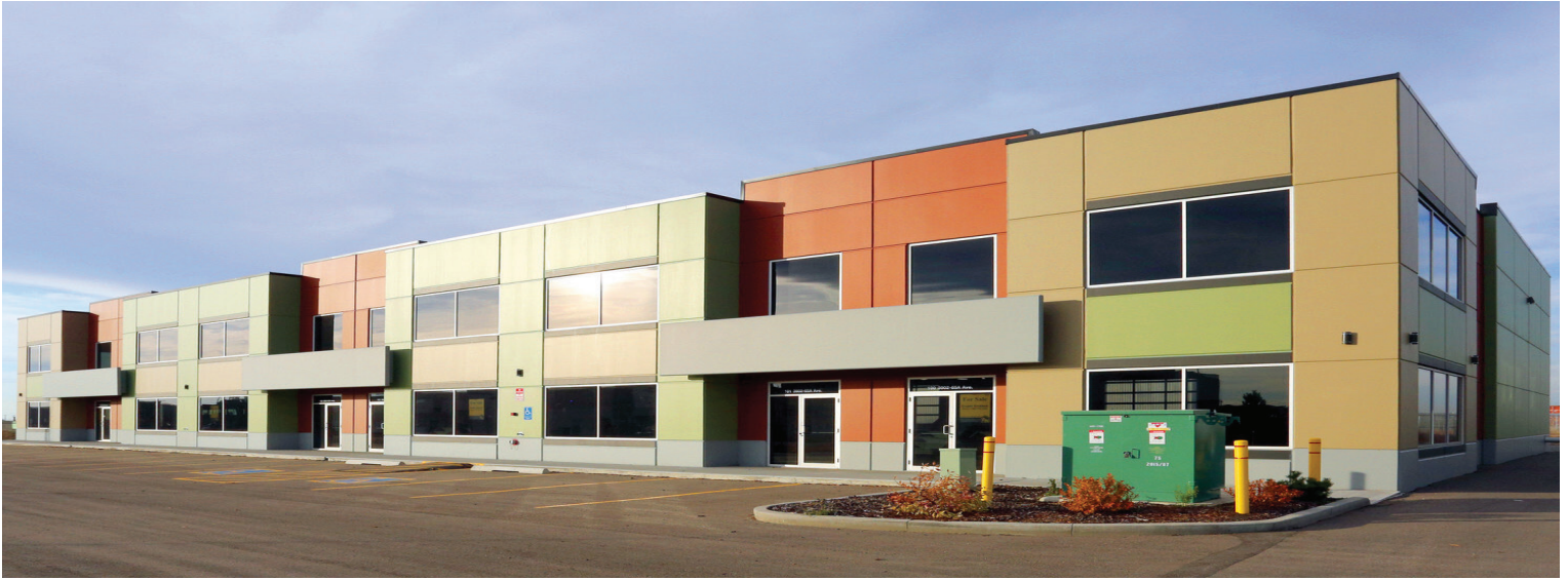
Overview of property
